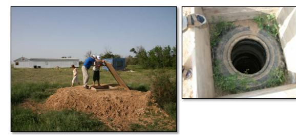
Underground storage tank of snowmelt water for drip irrigation. The meltwater forms a sweet water lens on top of the brakkish groundwater.
