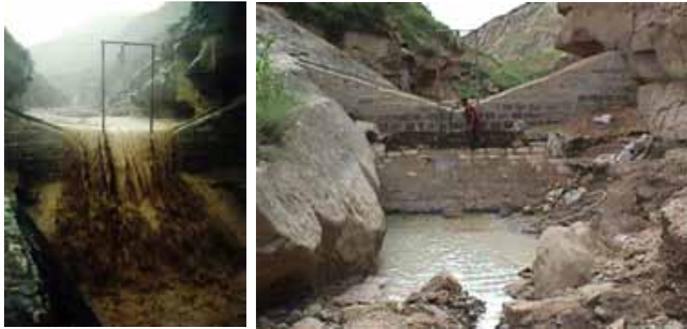
Figure 8.3. Large sharp crested weir (wall with steel knife top) to measure catchment discharge with ultrasonic level measurement. Although an ephemeral stream, construction of a flume was no feasible so a flat weir was chosen as design. (photo Erochina project ALTERRA).
