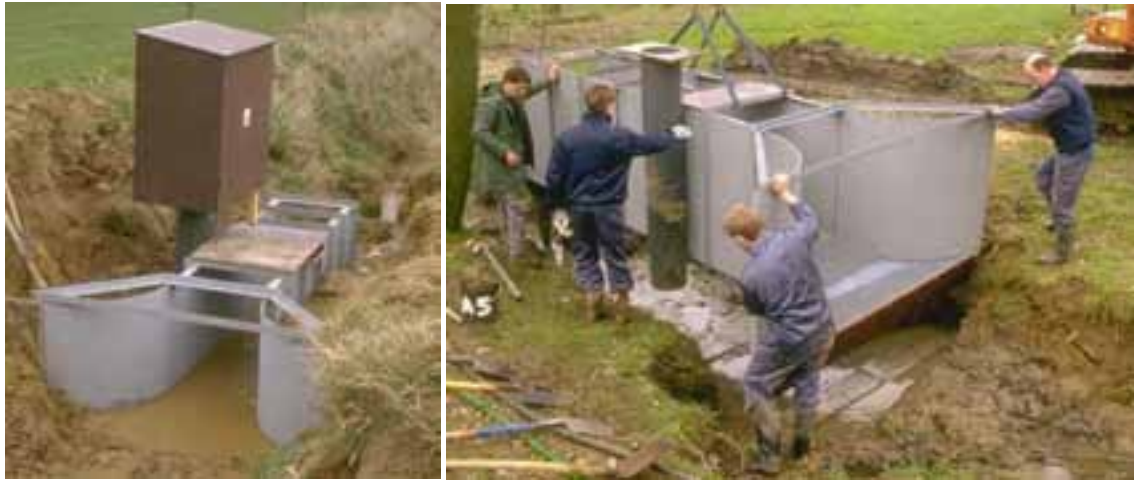
Figure 8.5. Placement of catchment level flume with stilling well (photos Physical and Regional Geography Research Group, K.U.Leuven).
