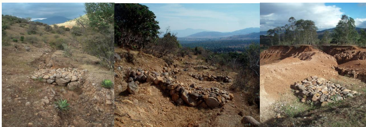
Examples of dams in gullies in EL Calabozo-Potrerrillos catchment (photos C. Prat, 2010)
