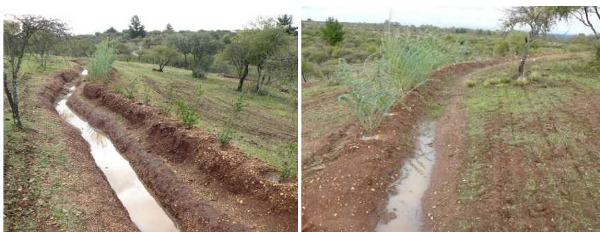
System of multiple purpose planting trees planting on infiltration trenches( left)
