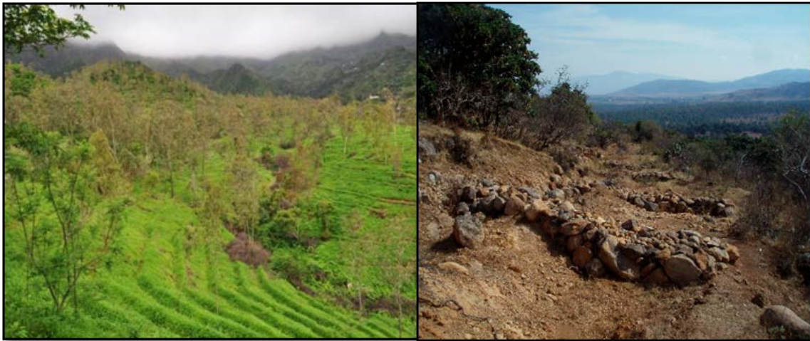
Figure 2.3.2. (left) Vegetative barrier helps make terraces in Cape Verde; (right) Construction of check dams in Mexico
