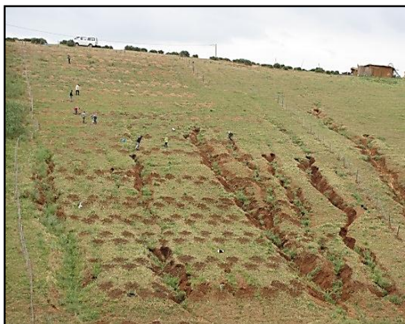
Morocco: gully stabilization with Atriplex
